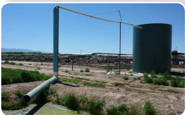
Example of an anaerobic digester on a CAFO. Photo courtesy of USDA.
